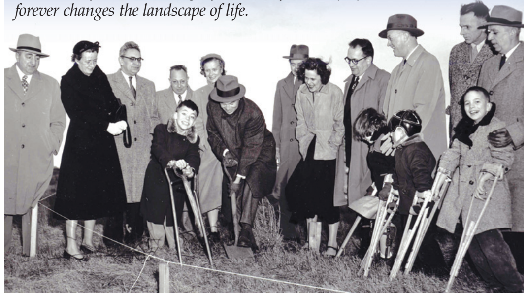
In 1954, Chuck Matheny helps break ground for construction of Matheny's new facility in Peapack.
